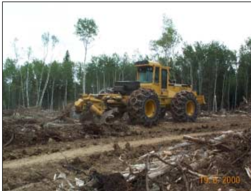
Figure 5.3 Site preparation equipment - power disc trencher mounted on a skidder.
