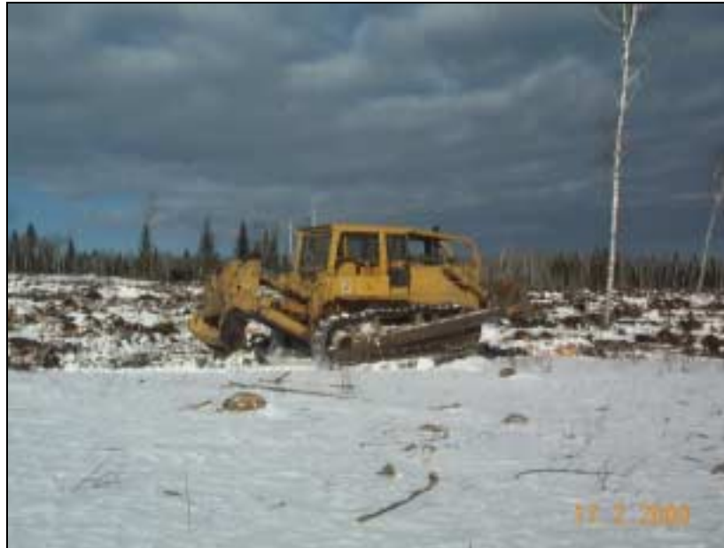
Figure 5.2 Site preparation equipment - ripper tooth plow mounted on a dozer.
