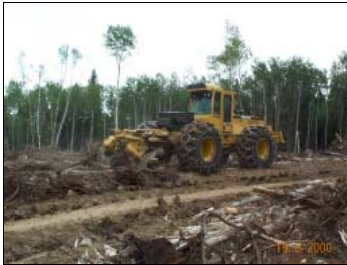
Figure 5.2 Site preparation equipment - power disc trencher mounted on a skidder.
