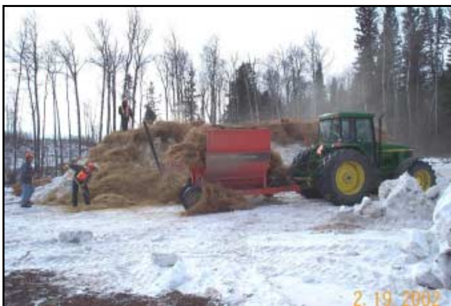
Figure 5.6 A snow cache in progress. Flax straw is being placed over one metre of clean snow.
