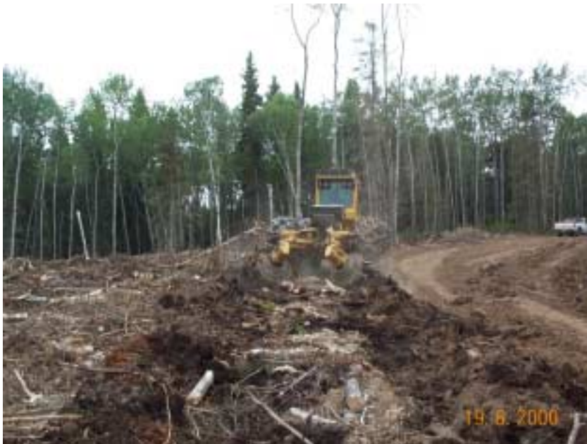
Figure 4.3 Site preparation equipment - power disc trencher mounted on a skidder.
