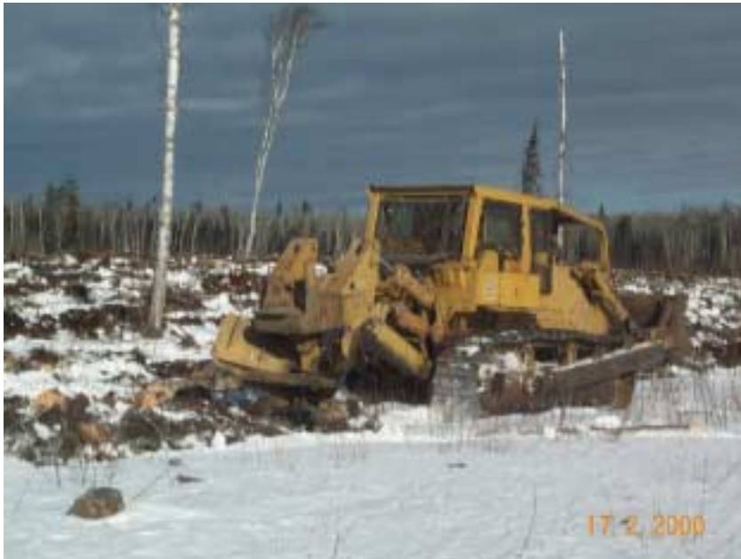
Figure 4.2 Site preparation equipment - ripper tooth plow mounted on a dozer.
